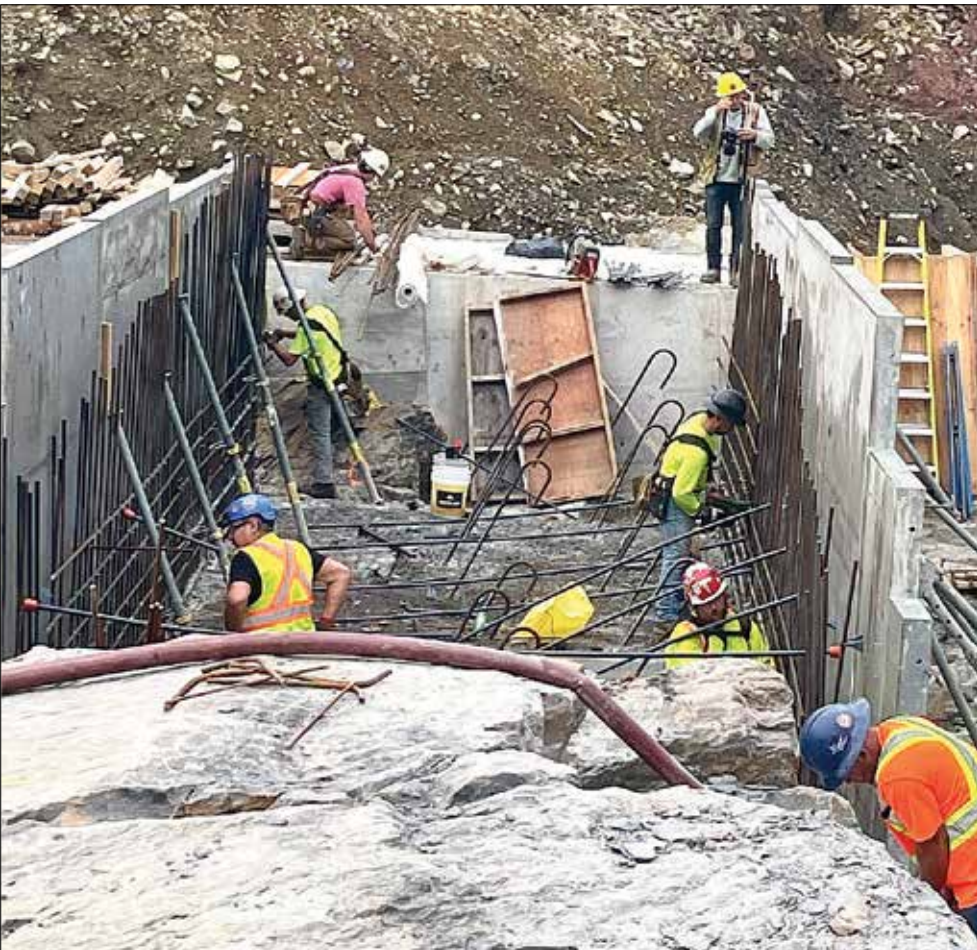
Specialized teams of ironworkers prepare the mesh grid of steel rebar inside the spillway trench at the construction site of the new Williams Lake dam in the Shaw Wilderness Park Photo: Cathy Vaughan, August 2026
