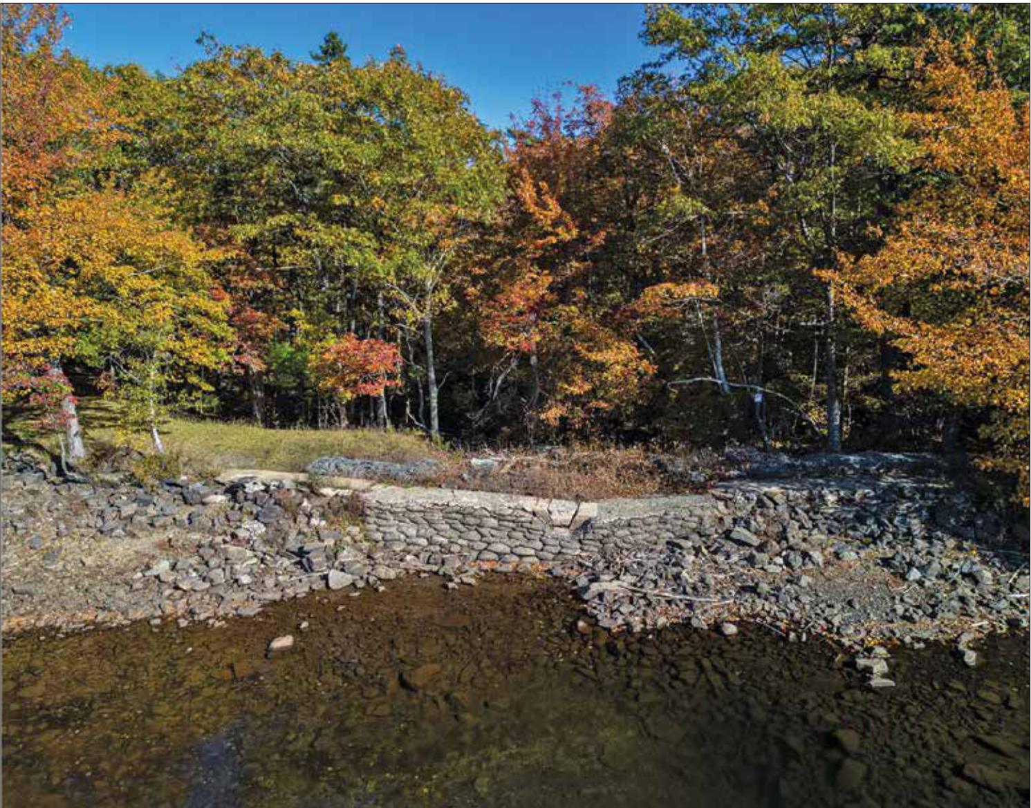
Photo: Build Nova Scotia, Williams Lake Dam.
