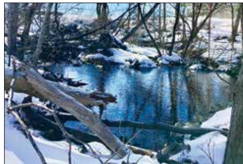
Lake water leaking under the Williams Lake dam, February 2025. Photo: Cathy Vaughan
