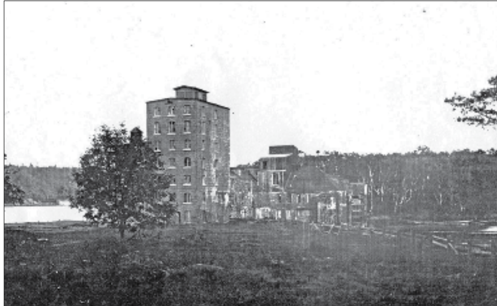
The photograph is of the Atlantic Sugar Refinery, in about 1929. Behind it is the Old Mill building which was burned in the 1912 forest fire on the Northwest Arm at Mill Cove. Photo courtesy Mainland South Heritage Society.
